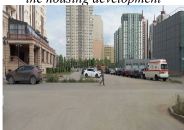
Photo 20. Increase of asphalt-concrete surfaces
