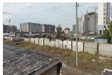
Photo 7. Construction of social infrastructure facilities
