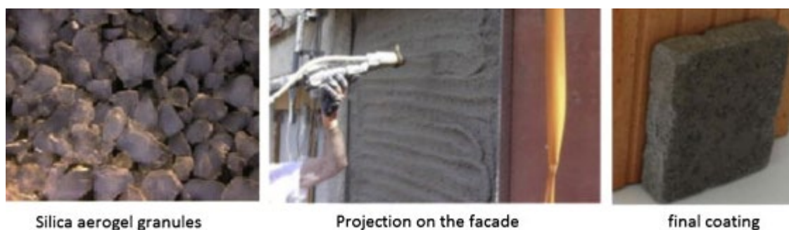
Figure 9 - Coating based on silica aerogel (Ibrahim et al., 2014).
