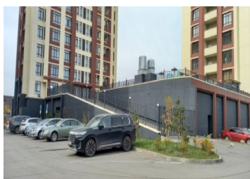
Photo 18. Underground space is not used
