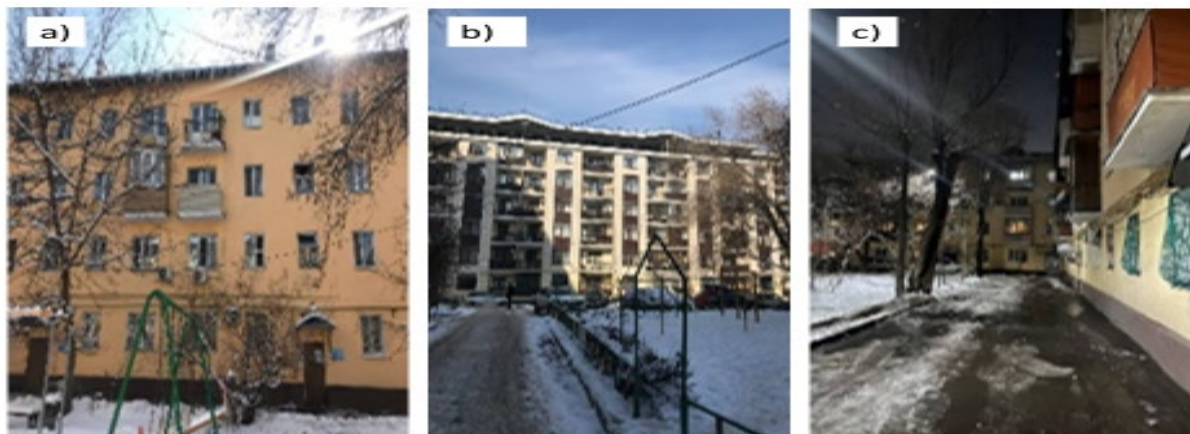
Figure 1 – Results compliance with the principles of "space protection, "eyes on the street": (a, b) Buildings of various ages; (c) Orientation of windows in kitchens and common rooms, exits to the courtyard (authors' materials).
