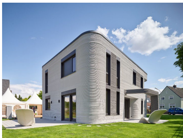
Figure 3 – The first residential house created with 3D printing in Germany, 2020. URL: https://habrastorage.org/getpro/habr/upload_files/412/d91/493/412d91493671aaebd2e8feb6079713ab.jpg
