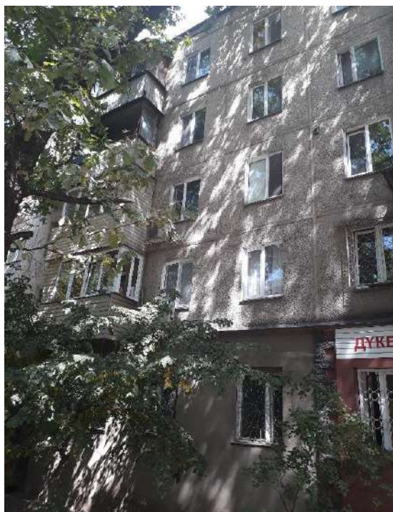
Figure 1 – Large-panel building with a flexible first floor, Mynbayev str.47 (author's material)
