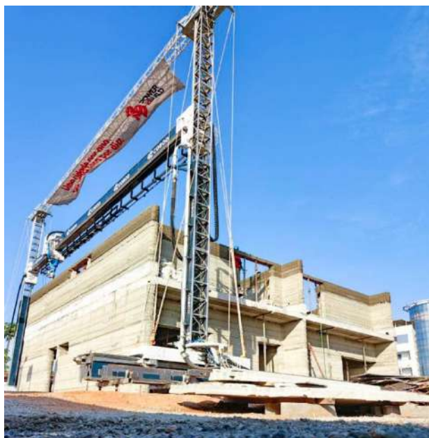
Figure 3 – Construction process of the residential duplex implemented using 3D-printing technology in Angola. Architect: Ilídio Daio, Power2Build (Pineiro, A. 2025).
