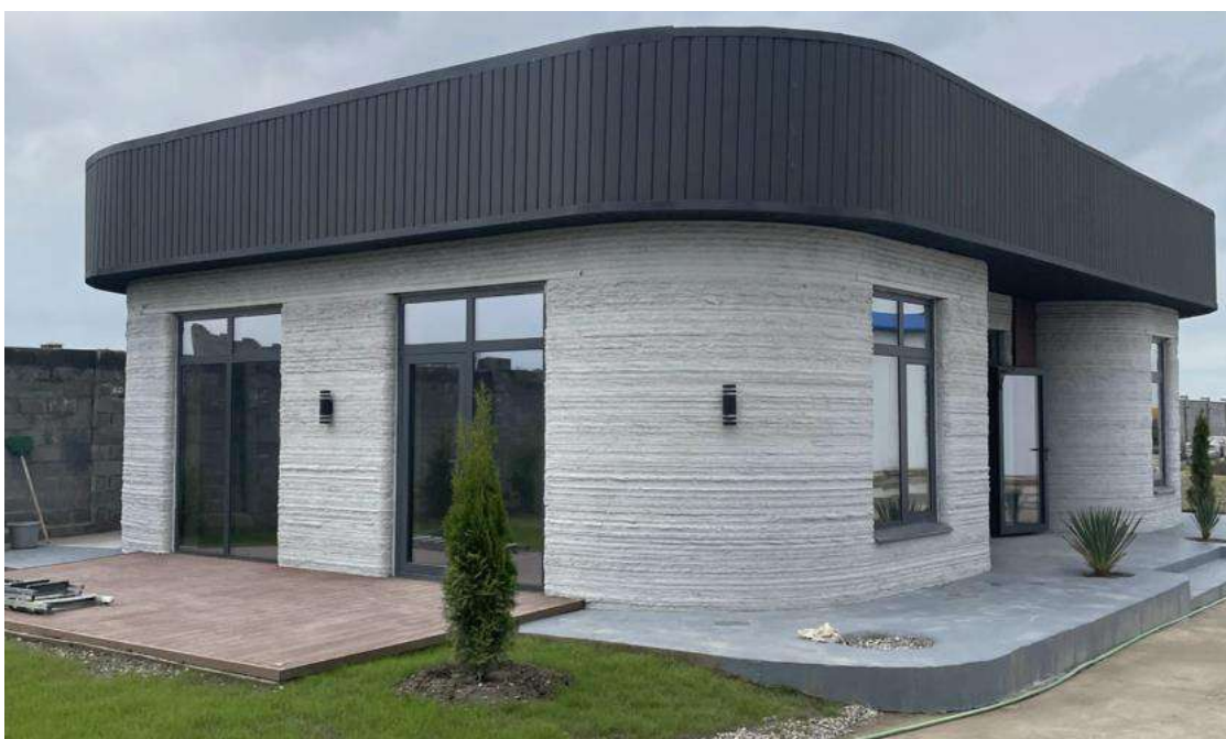
Figure 4 – The first residential building in Central Asia constructed with a COBOD BOD2 3D printer. Architect/Builder: BM Partners 3D Print (authors' material).
