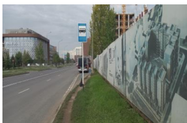
Photo 11. Pedestrian accessibility and station condition
