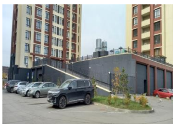
Photo 18. Underground space is not used
