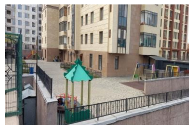
Photo 13. Adjacent area to the residential complex
