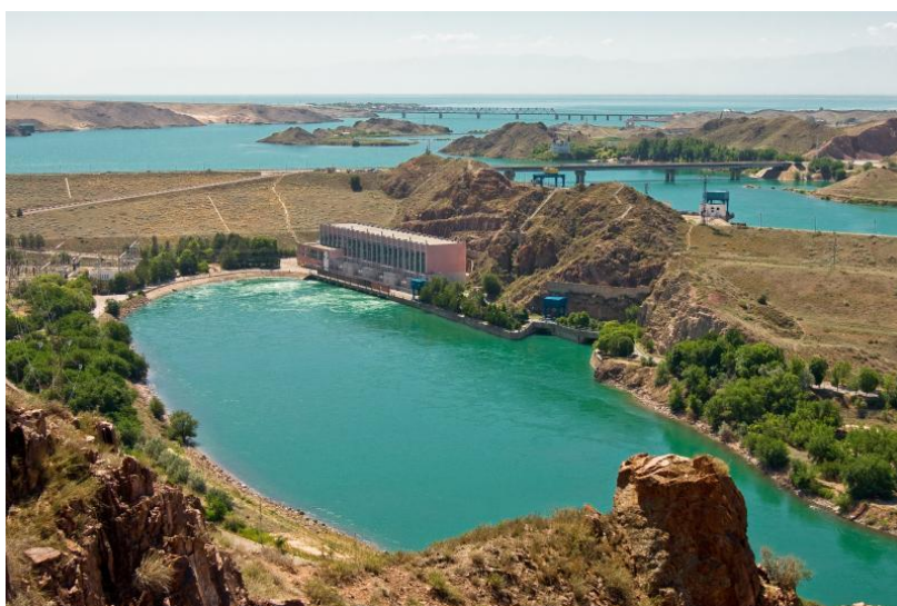
Figure 1 - General view of the Sh. Chokin Kapchagay HPP: powerhouse and tailrace channel, looking downstream along the Ili River [from open sources]
