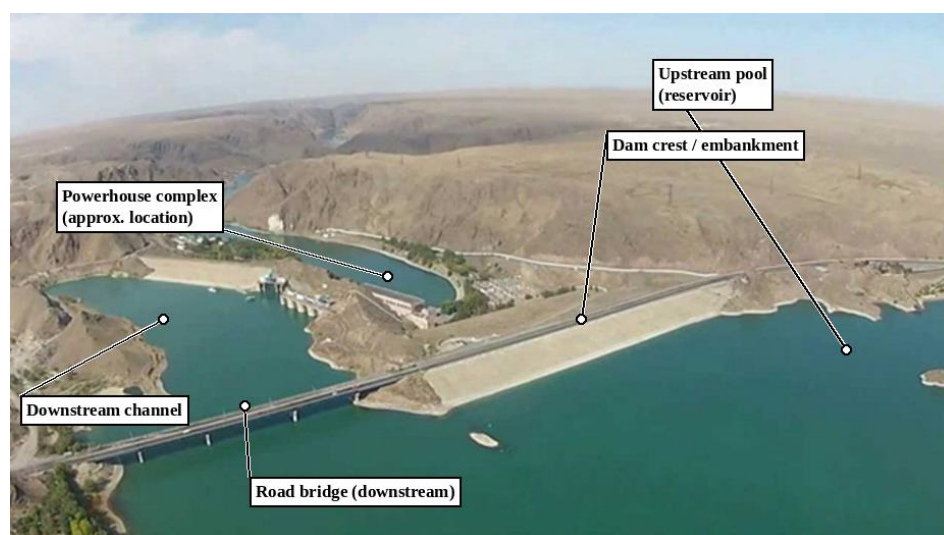
Figure 2 - Aerial view of the Kapchagay HPP hydraulic complex and its general structural layout [Author's material]
