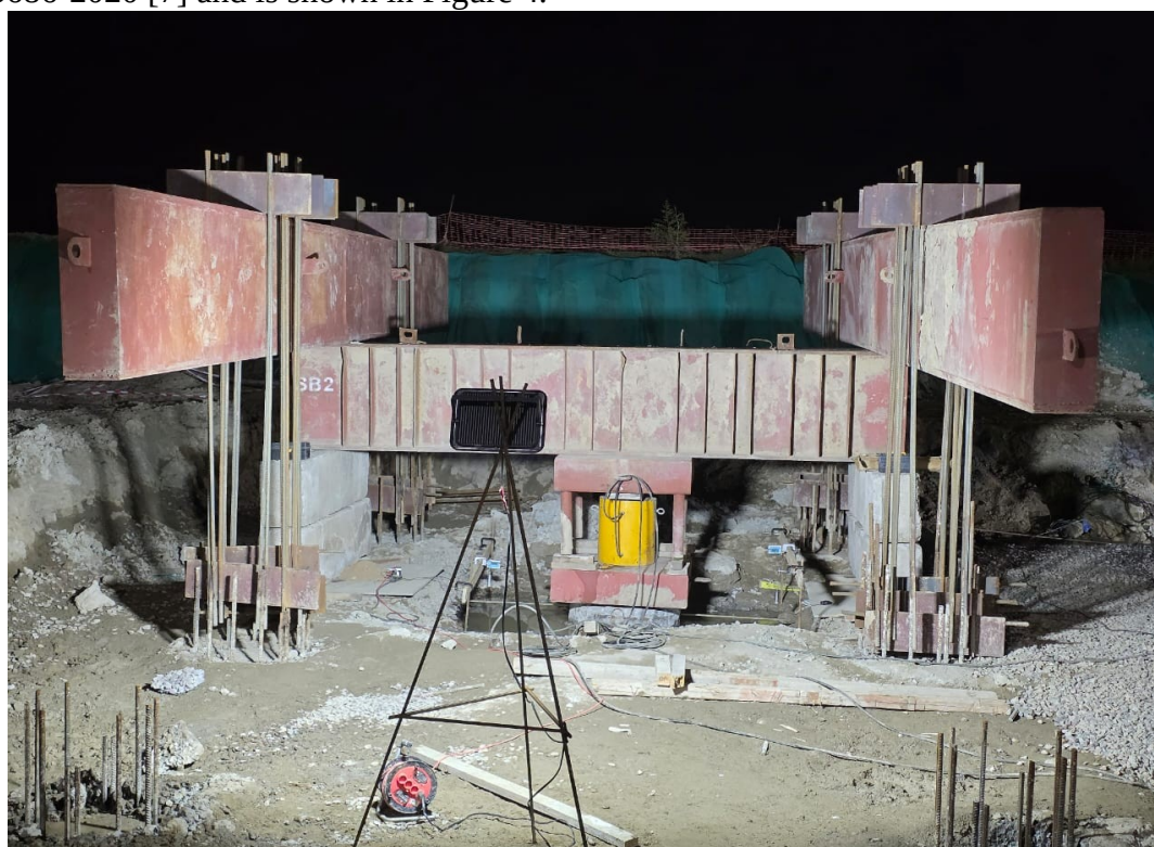
Figure 4 - Loading platform for static testing of a bored pile [Authors' material]
