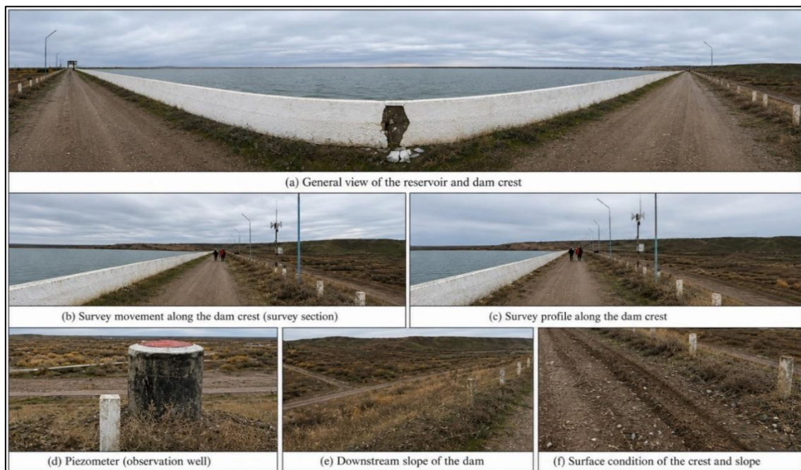
Figure 3 - Field conditions of the Tasotkel dam and the GPR survey environment: (a) general view of the reservoir and dam crest; (b-c) survey movement and profile layout along the crest; (d) piezometer (observation well); (e-f) downstream slope and surface condition of the embankment (author’s materials)
