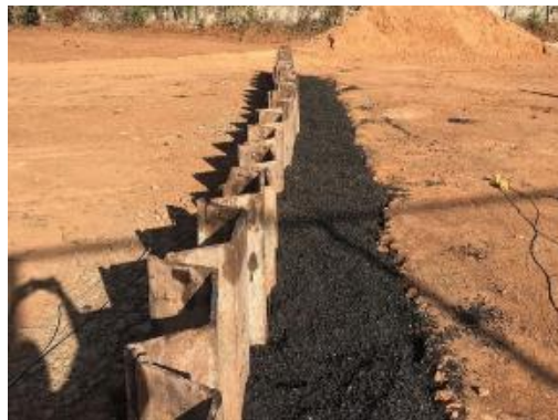
Figure 2 - Field installation view of a vibration-isolation trench barrier filled with a rubber-soil composite mixture (author's material)
