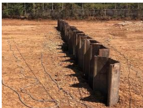
Figure 1 - Experimental installation of a steel vibration barrier for limiting wave propagation in the soil mass (author's material)
