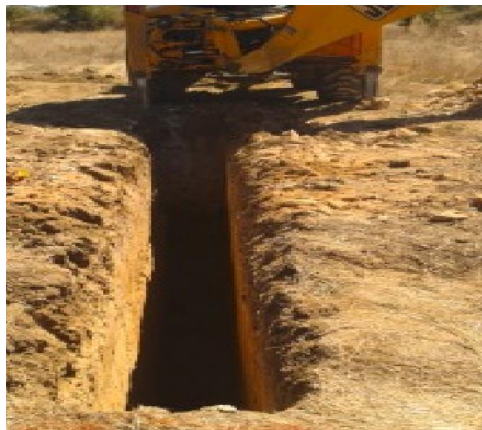
Figure 4 - Mechanized excavation process of a trench designed to limit the propagation of vibration waves (author's material)
