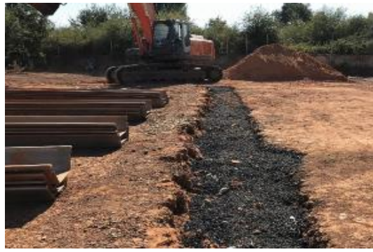
Figure 3 - Construction stage of the installation of a trench barrier designed to attenuate railway-induced Vibrations (author's material)
