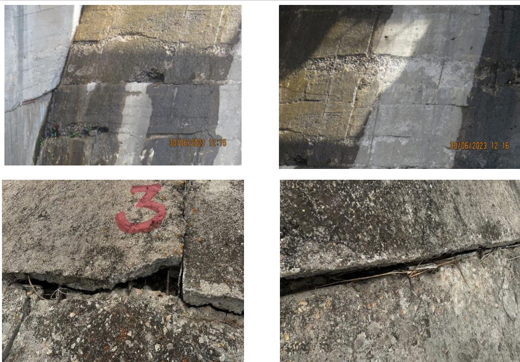
Figure 2 – Inspection fragments showing cracking and opening of joints in the deteriorated area. (author's materials)
