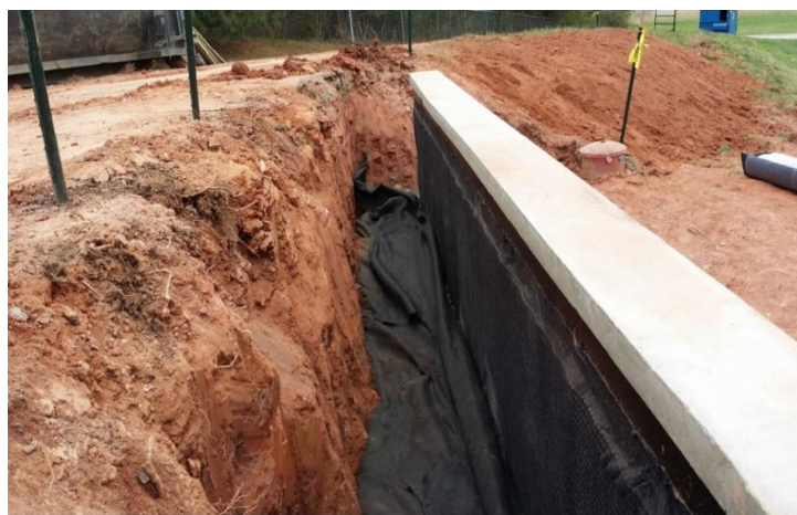
Figure 4 - Geotextile under the foundation (catalogue Baurex, 2024)
