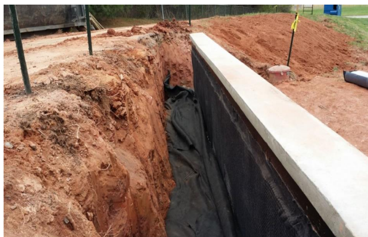
Figure 4 - Geotextile under the foundation (catalogue Baurex, 2024)
