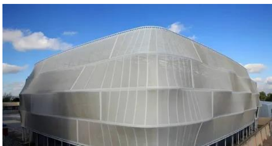
Figure 3 – Fiberglass architectural membrane (Milanchik's library, 2025)
