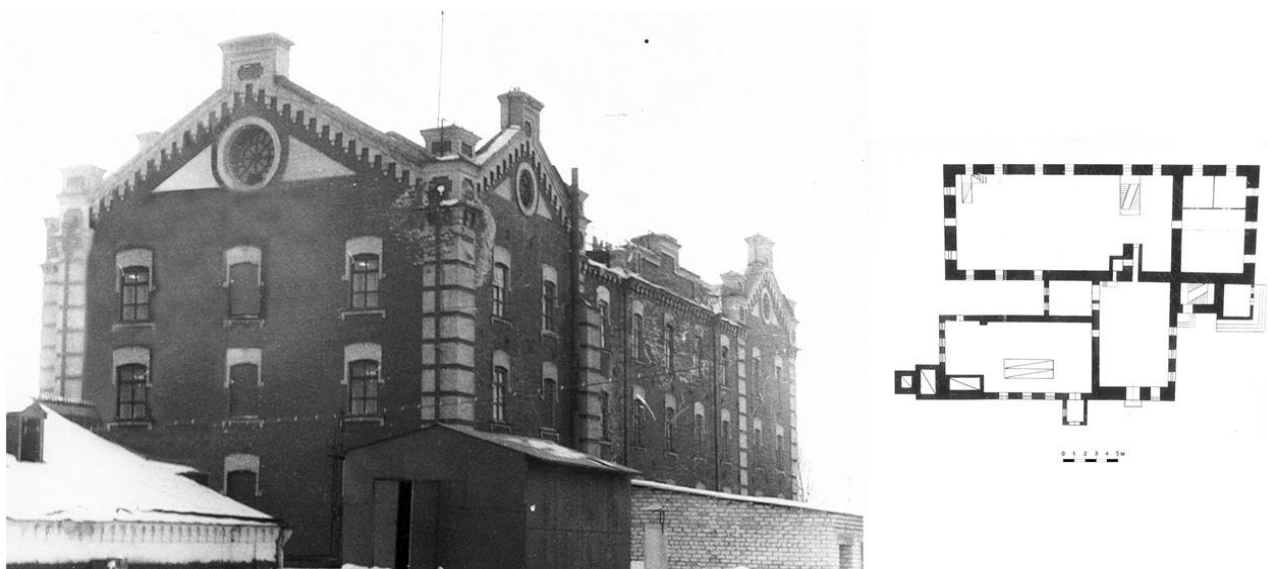
Figure 2 – Hardware and fittings factory building (formerly Musin’s merchant mill), general view and plan (author’s material)
