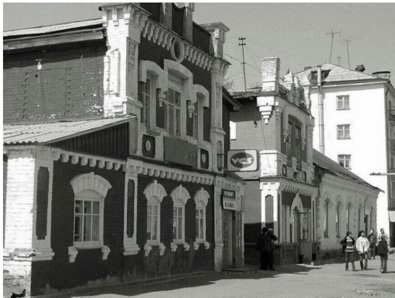
Figure 4 – Buildings of the mechanical workshops of O.F. Kostyurin (author's material)
