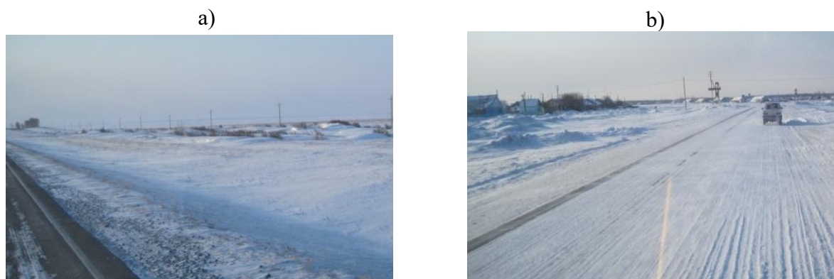
Figure 4 – Snow and ice formations on the pavement surface of the Kostanay-Surgan highway a – snow cover, section km 40–82; b – snow pack, section km 89–103 (author's materials)
