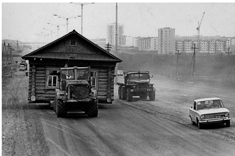
Figure 2 – Transportation of an assembled log house (Bevzenko, 2018)
