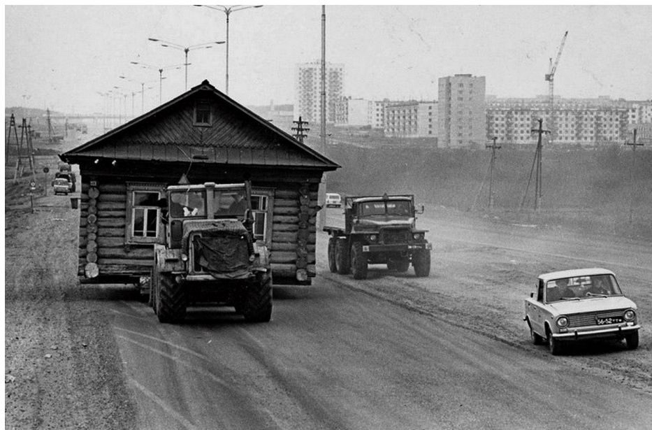
Figure 2 – Transportation of an assembled log house (Bevzenko, 2018)
