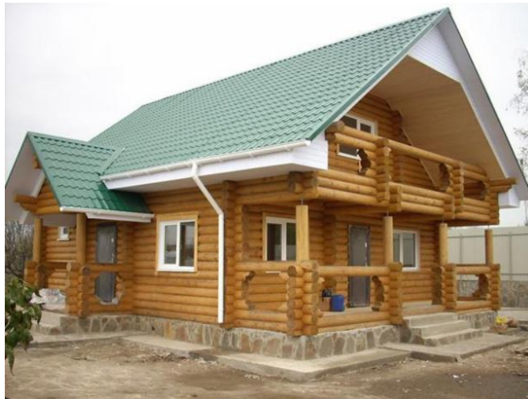
Figure 1 – Wooden house, manufactured in a factory and assembled on site from individual elements (Bevzenko, 2018)
