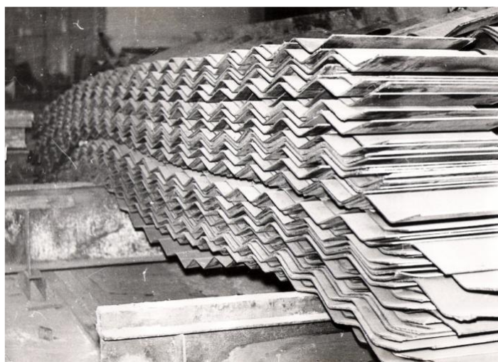
Figure 2 – Corrugated webs in the assembly shop.
