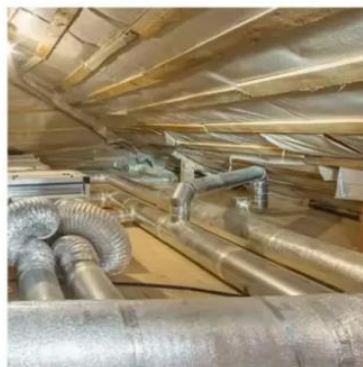
Figure 10 - Example of a HVAC system insulation with reflective multi-foil (Lee et al., 2016).
