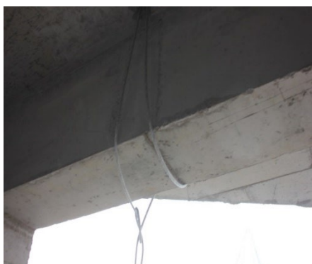
Figure 5 - Cable attachment to building structures (author's materials)
