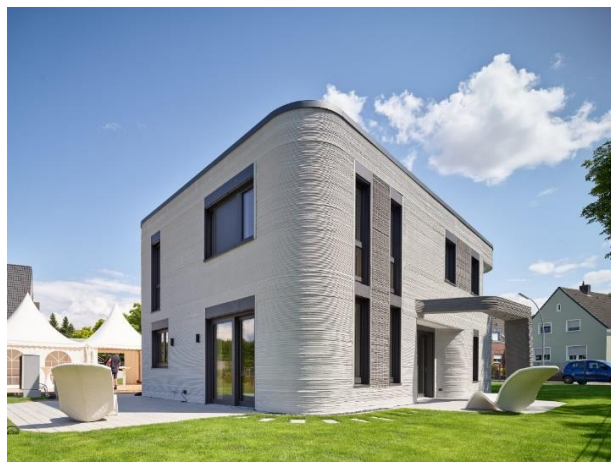
Figure 3 – The first residential house created with 3D printing in Germany, 2020. URL: https://habrastorage.org/getpro/habr/upload_files/412/d91/493/412d91493671aaebd2e8feb6079713ab.jpg
